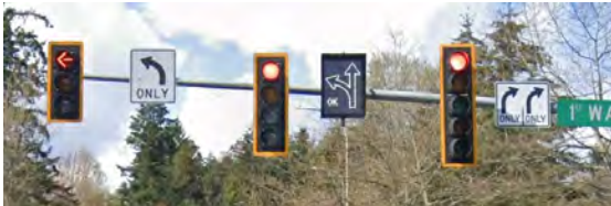
Figure 12. Variable turn sign at S 336th St and 1st Way S
